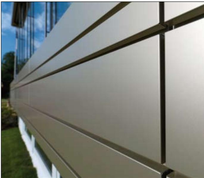
*Zinc-magnesium coating and four paint coats ensure long-lasting quality.*
