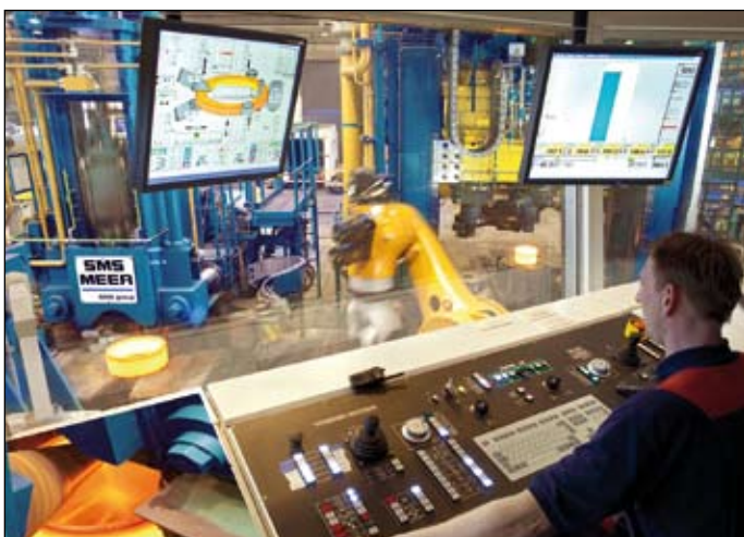
The new RiWa 2000/80 ring rolling plant must increase the annual capacity of the Ovako works to 55,000 t. Photo courtesy of SMS Meer
