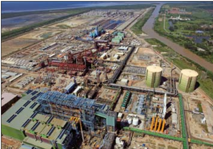
With total investment €5.2 billion, the iron and steel mill is the first major steel mill to be built in Brazil since the mid-1980s. Photo courtesy of ThyssenKrupp
