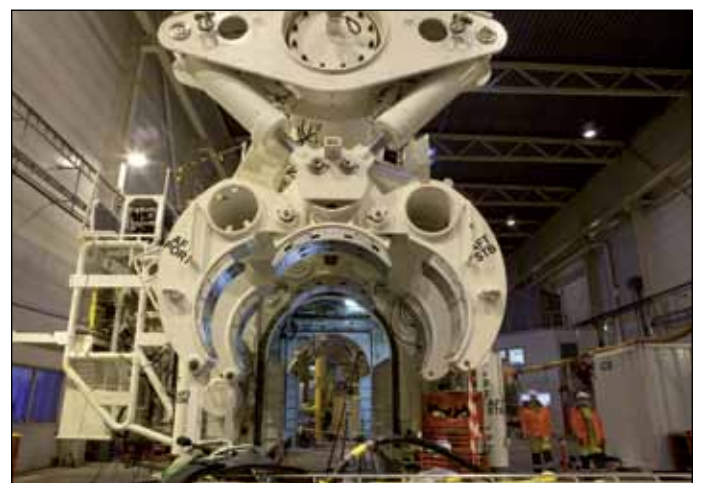
The welding habitat is a dry environment where divers work without diving equipment to set up the automatic welding machine. The welding is completely controlled from the dive support vessel.
